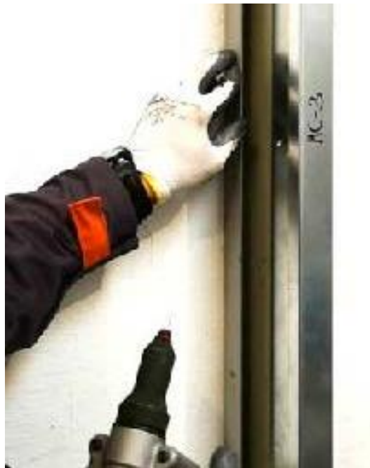
Figure 15. Clamp profiles for jambs.
