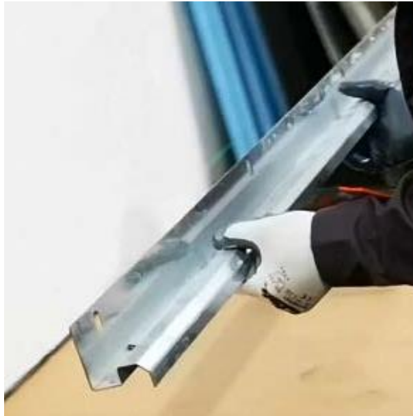
Figure 8. Horizontal starting profile of the system.
