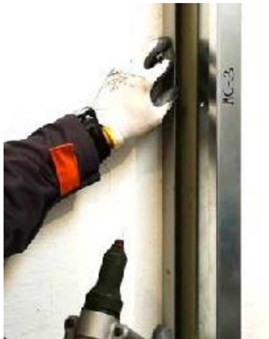
Figure 23. Clamp profiles for jambs
