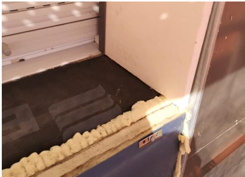
Figure 32. Insulation and waterproofing layer on a window perimeter
