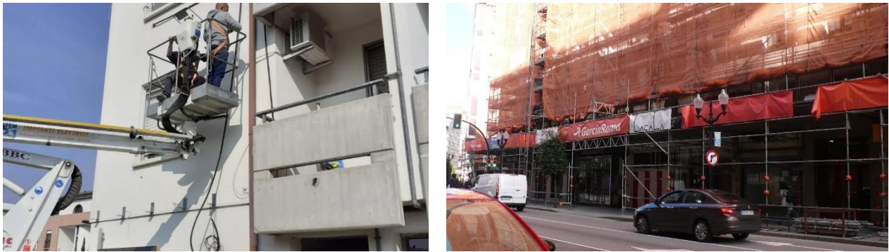
Figure 40. Crane platform and scaffolding installation system
