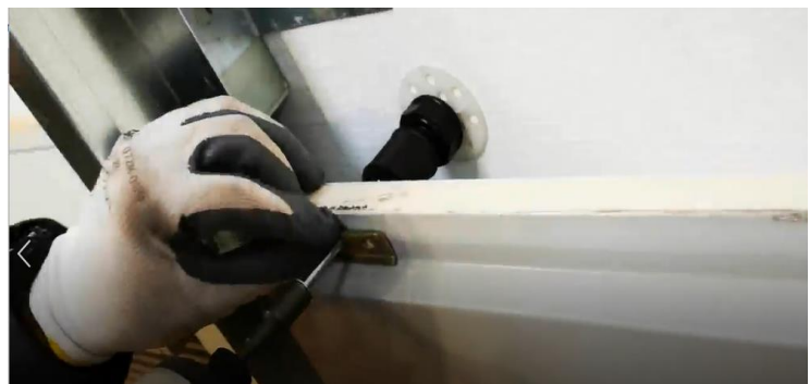
Figure 43. Demonstration of insulating panel installation
