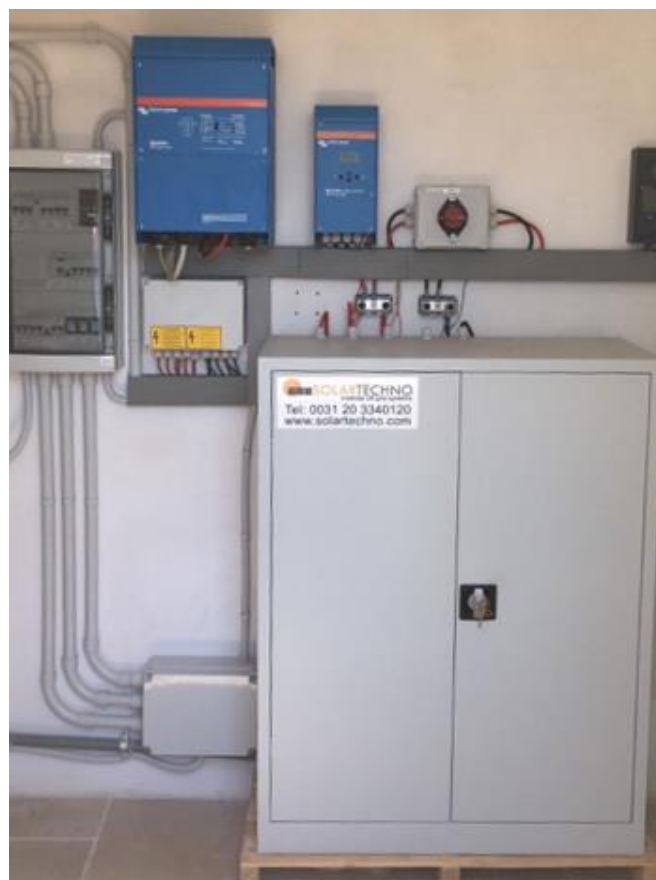
Figure 28. Example of battery enclosure with inverters, battery charges, AC junction box
