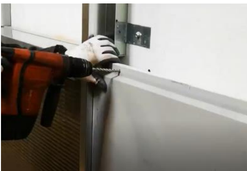
Figure 46. Demonstration of insulating panel installation
