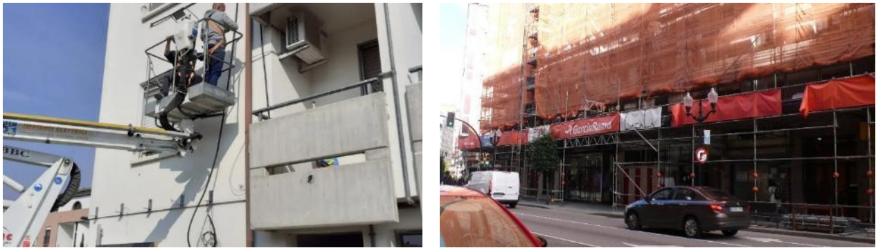
Figure 43. Crane platform and scaffolding installation system
